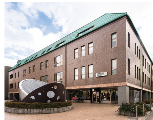
▲ Building No.27 (Azusa Ono Commemorative Building)
