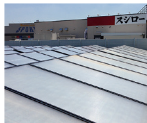
▲ Hybrid heat-source system using solar heat and ground-source heat at Honjo Smart Energy Town
