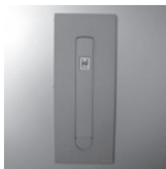
Figure 1-4-11. The smoke ventilation window switch
