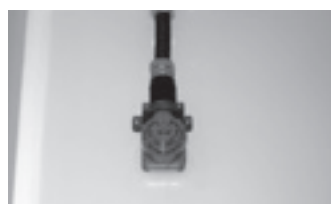
Hydrogen and acetylene sensor
