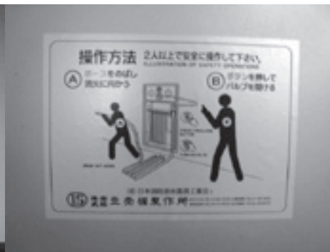
Figure 1-4-3. How to operate an indoor fire hydrant
