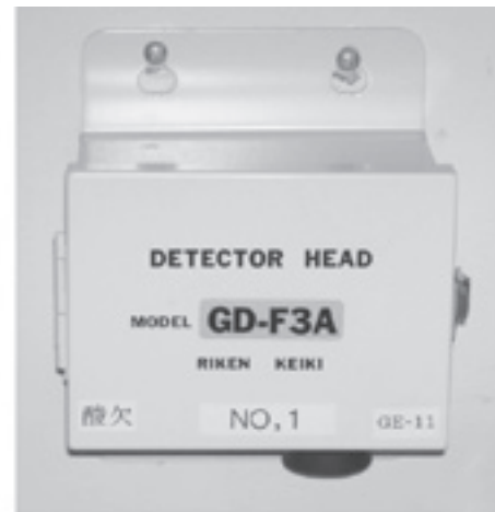
Oxygen sensor Set on wall in two locations
