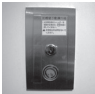
Figure 1-4-9. The operating panel of the smoke-proof hanging partition walls
