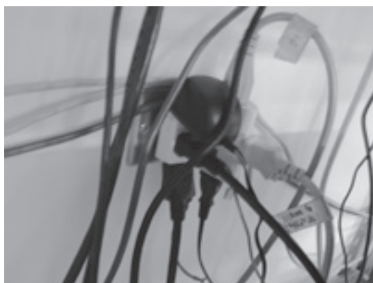
Figure 3-5-1. Octopus wiring caused by directly connecting a tap to the wall outlet
